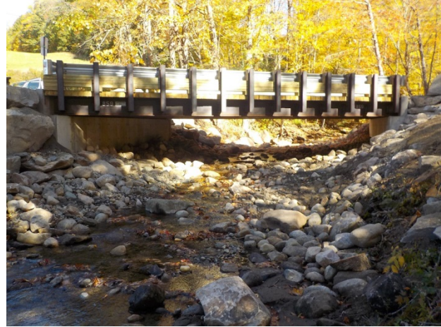
After – 40 foot span bridge installed summer 2016
