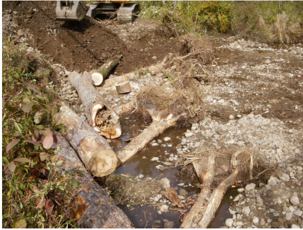
Large wood additions provide habitat and stabilize the eroding bank.
