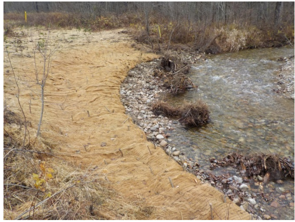
Post construction plantings; 291 willow stakes and speckled alders.
