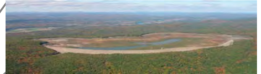
Northfield Mtn Pumped Storage
