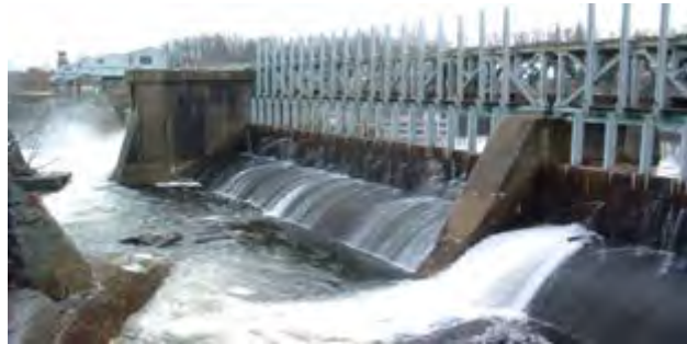
Bellows Falls Dam
