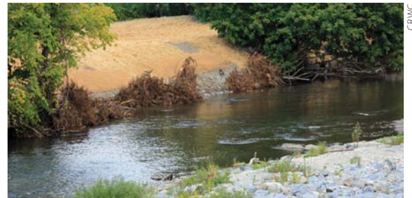
Root wads are a natural way to restore flood-eroded stream banks. Trees will be planted this year to further stabilize the bank & provide wildlife habitat.
