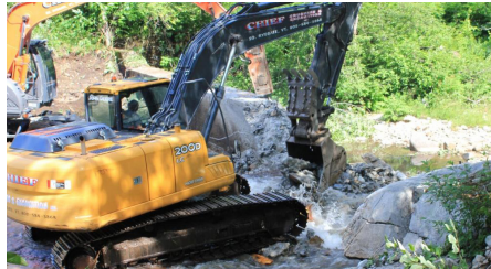
In July, CRWC and partners worked to remove the dam.
