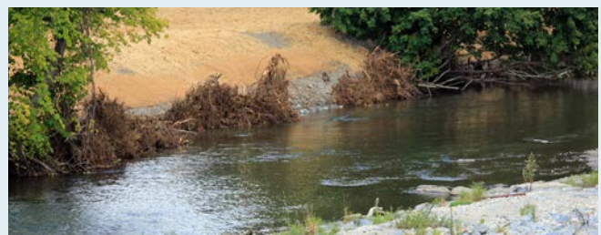
Root wads help stabilize the stream bank at the Bradford Golf Club in VT. Photo: CRWC
